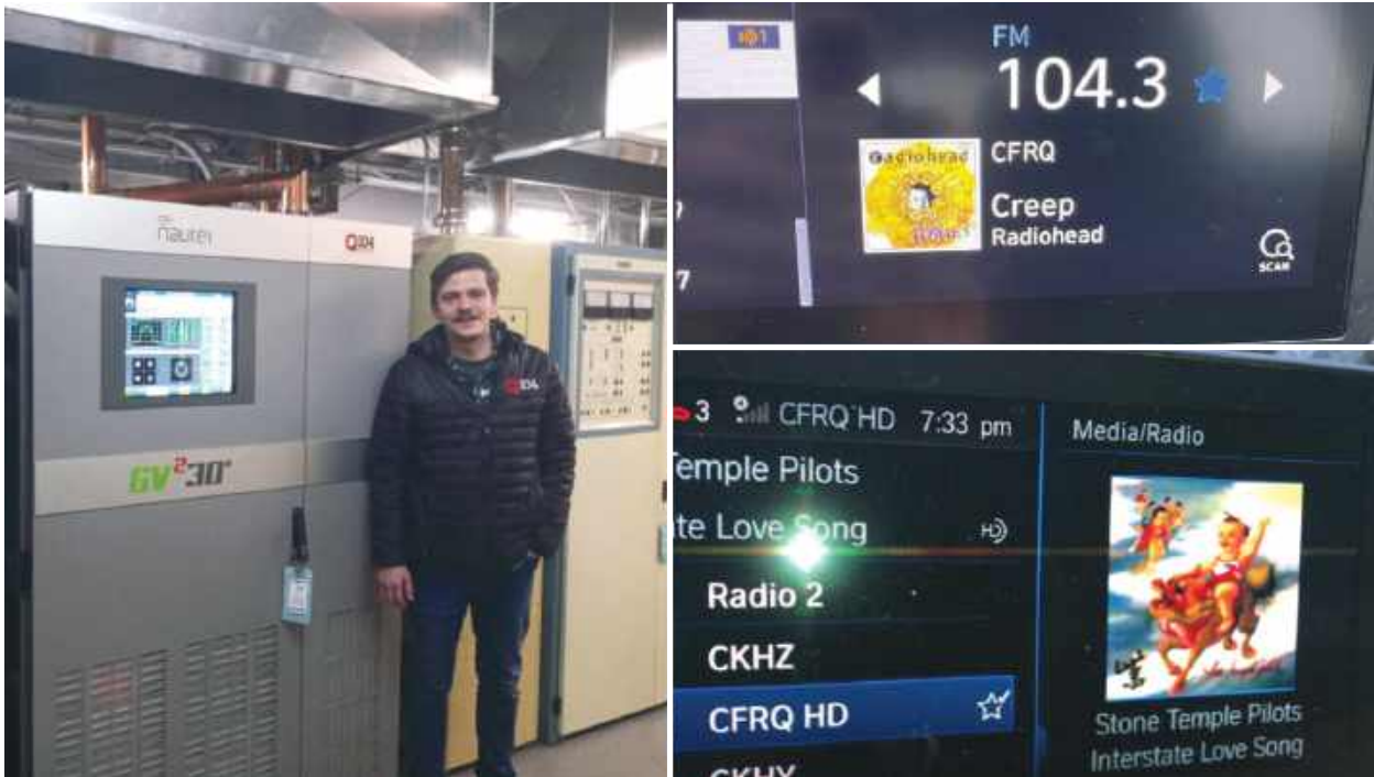
Left Stingray Group station CFRQ(FM) in Halifax, Nova Scotia, has installed the first GV2-30 transmitter and has adopted the software-based air chain approach. At left is Matthew Gillie, director of engineering in Nova Scotia.
