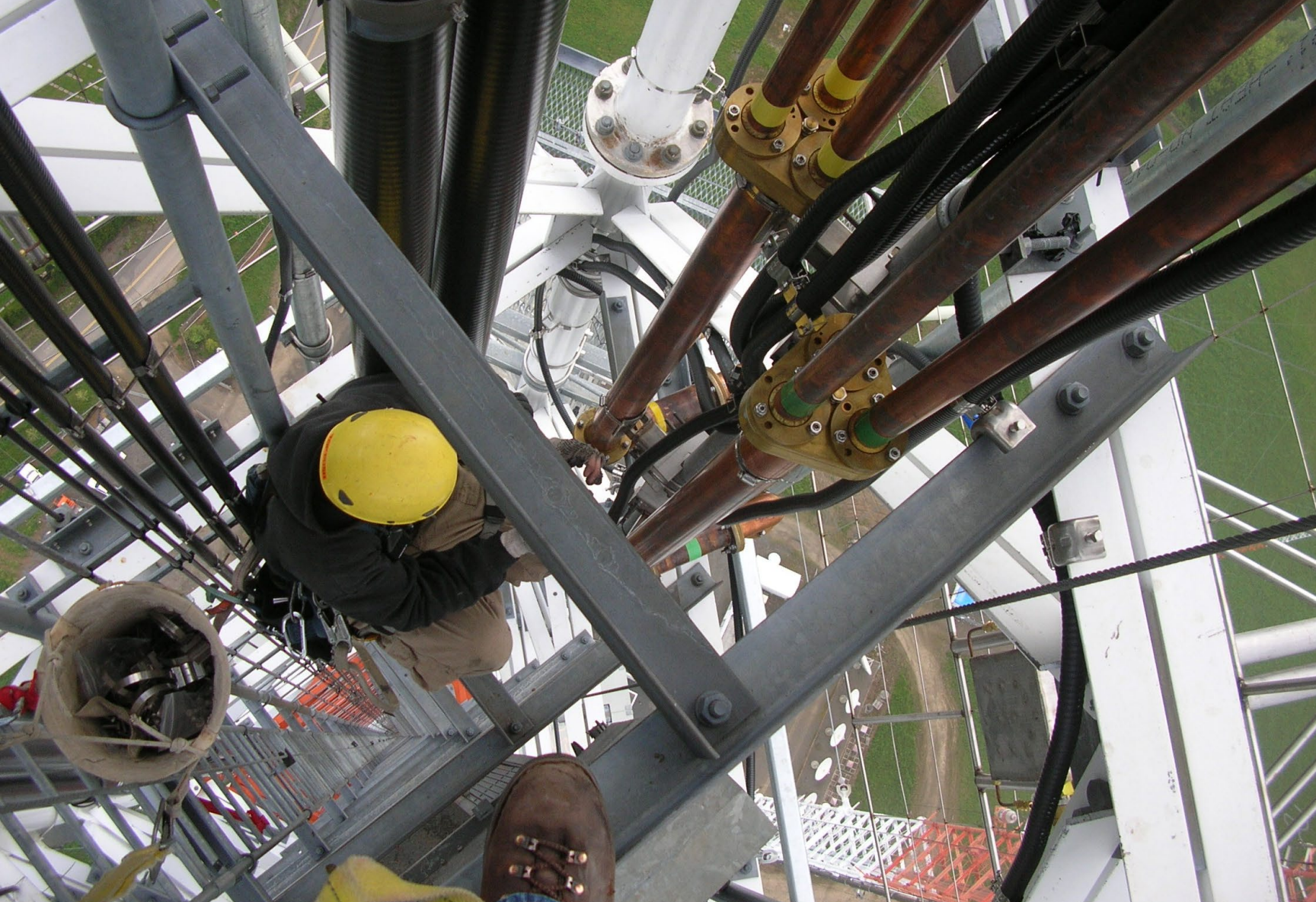
Above: Installation of coax hangers.
