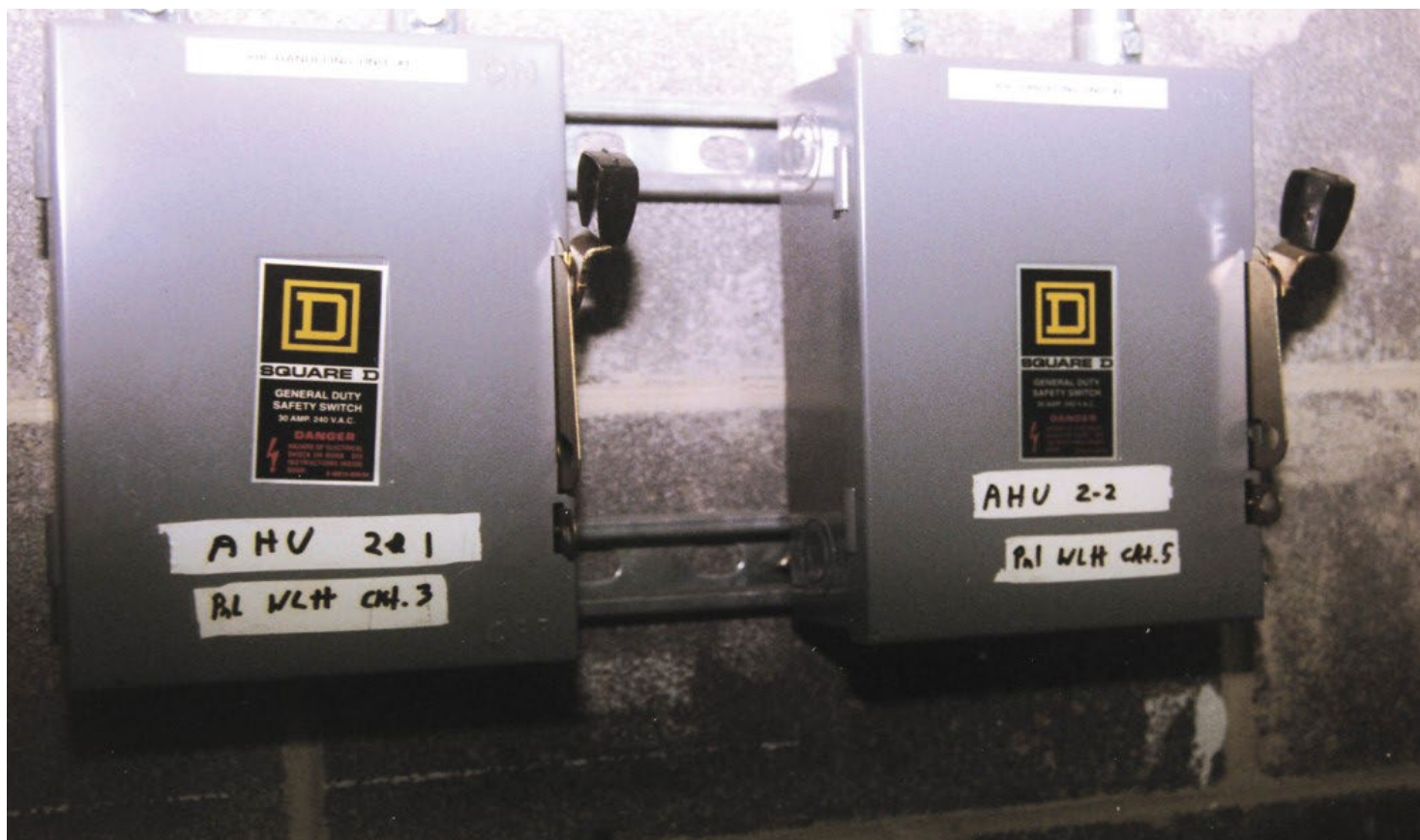
Above Fig. 12: Duct or gaffer's tape works just fine for identifying AC disconnects.
