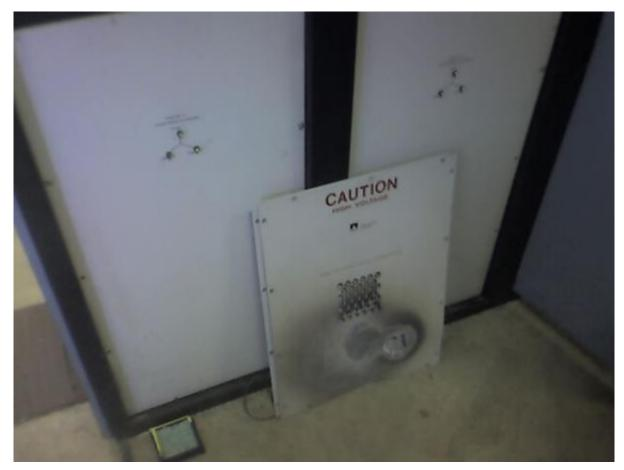
Poor airflow, or insufficient cooling, can be expensive!!!
