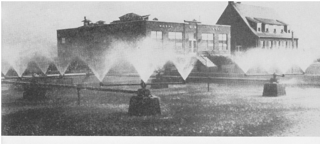
Fig 1 "The Fountain"-- Cooling spray pond at 500 kW WLW (1932)
