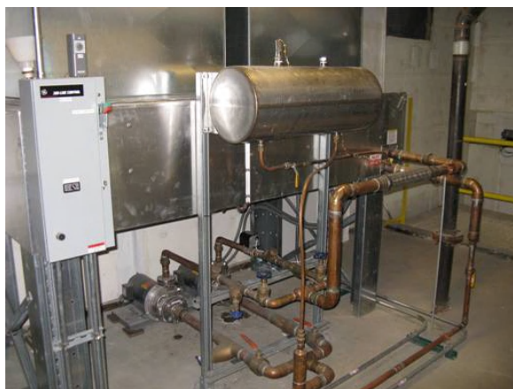
Fig. 5- Heat exchanger in Continental tube system (WNCL, Columbus, OH)
