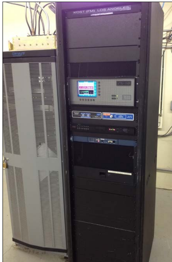
Translator equipment should be built into a locked cabinet to keep its operation secure.
