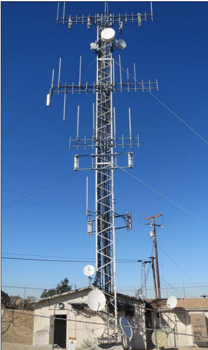
Shared sites pose many potential problems for translators. Input filtering for off-air reception will likely be needed in addition to output filtering.
