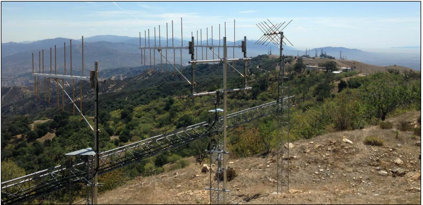
Translator antennas should get just as much consideration and expertise for their installation as would any other transmit antenna you install. Take care to allocate a sufficient amount in your budget to satisfy this need.
