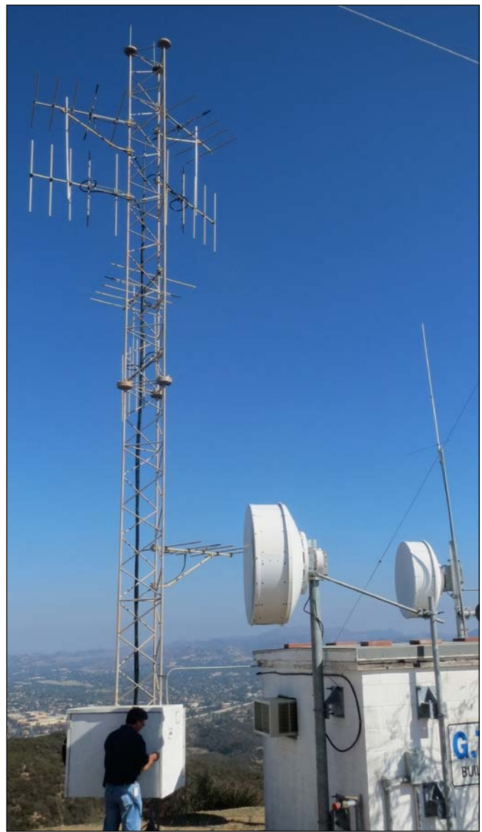
Translator antennas can be made up of “composite” patterns that include multiple elements. Try to keep them isolated from other antennas to minimize pattern distortion.
