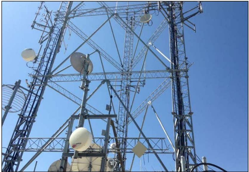
Shared communications sites such as this one are often supplied with good connectivity from Telco, thus providing another option for the delivery of programming.
