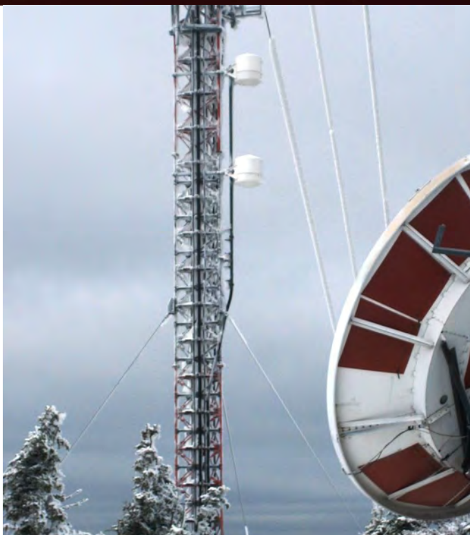
Directional FM antenna systems raise some particular questions. Shown is a Dielectric DCR-H system with radomes.
