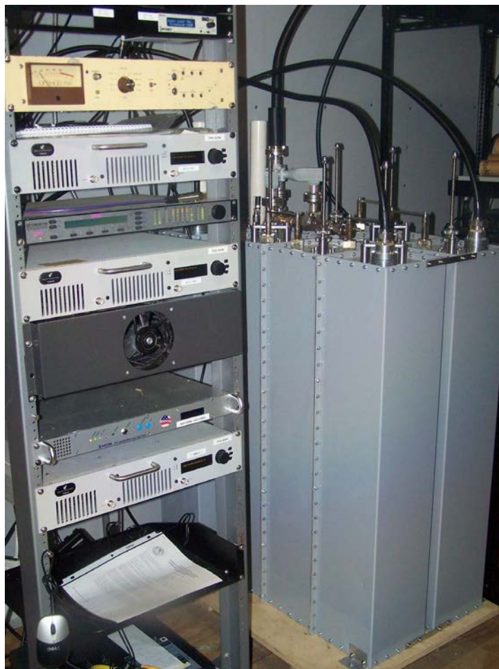
W240CP, W248CF and W281BV, all with 250 Watts and combined into an inexpensive two-bay broadband antenna at the top of the tower, prove excellent service to Bowling Green, Ky.
