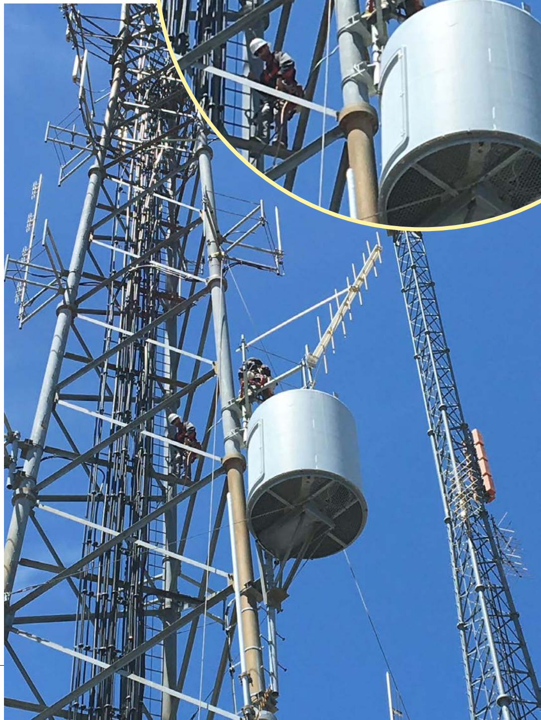
Tower workers install a directional translator antenna.
