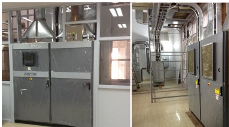
Old RCA BTF20E transmitters replaced with NVIt7.5's, NSW, Australia >
